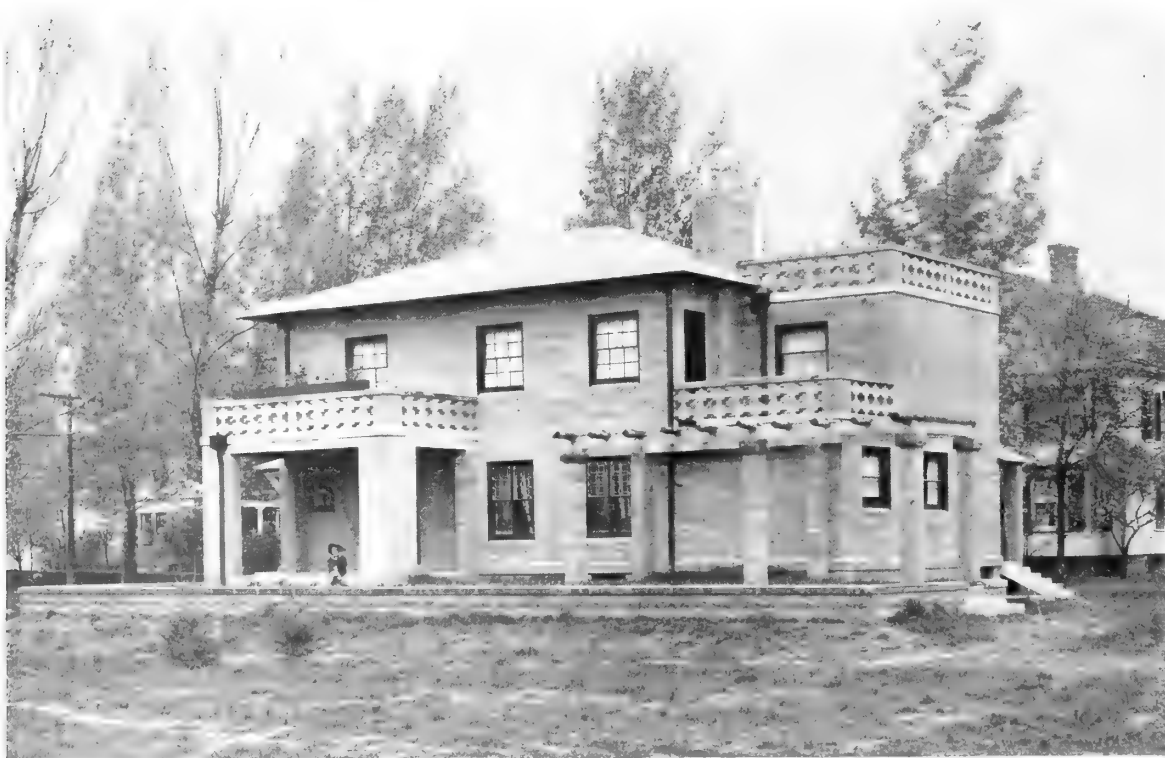
14—Skilled Labor is Not Required to Make the Hollow Concrete Block of Which the House is Built
